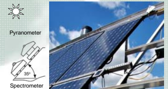
Fig. 3 (a) Outdoor PV performance and meteorological data monitoring system.
